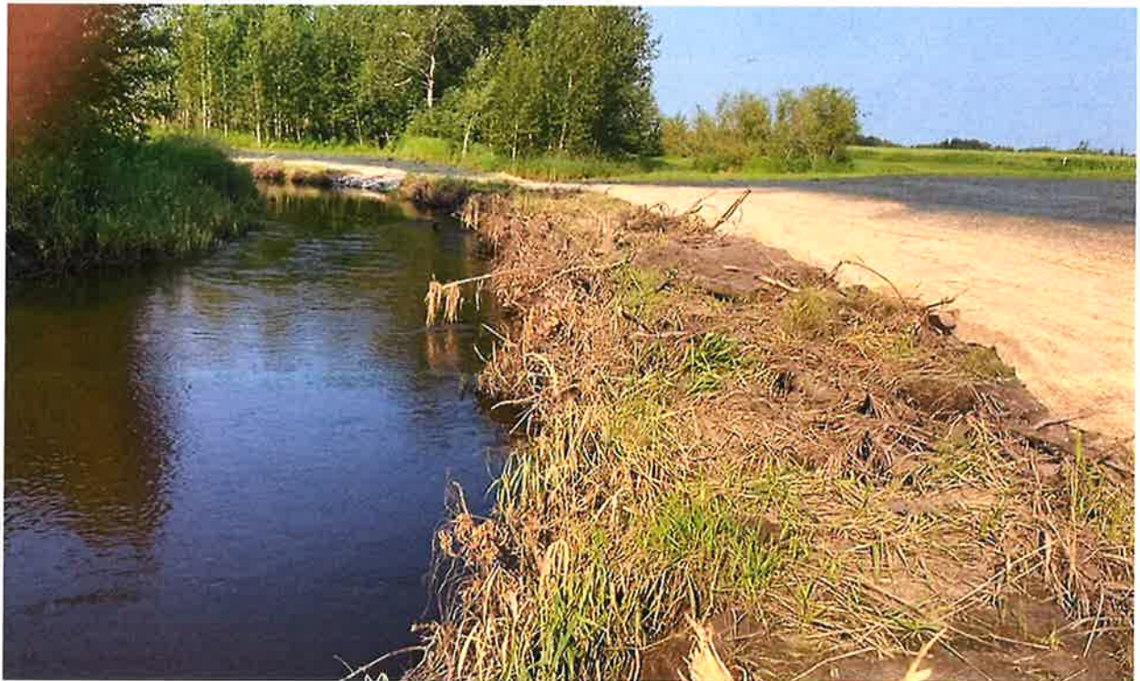
Above: Streambank stabilization project completed at the Victor Lundemo and Jason Eichenberger properties utilizing a combination of toe wood (root ball) and rip-rap methods of stabilization.
