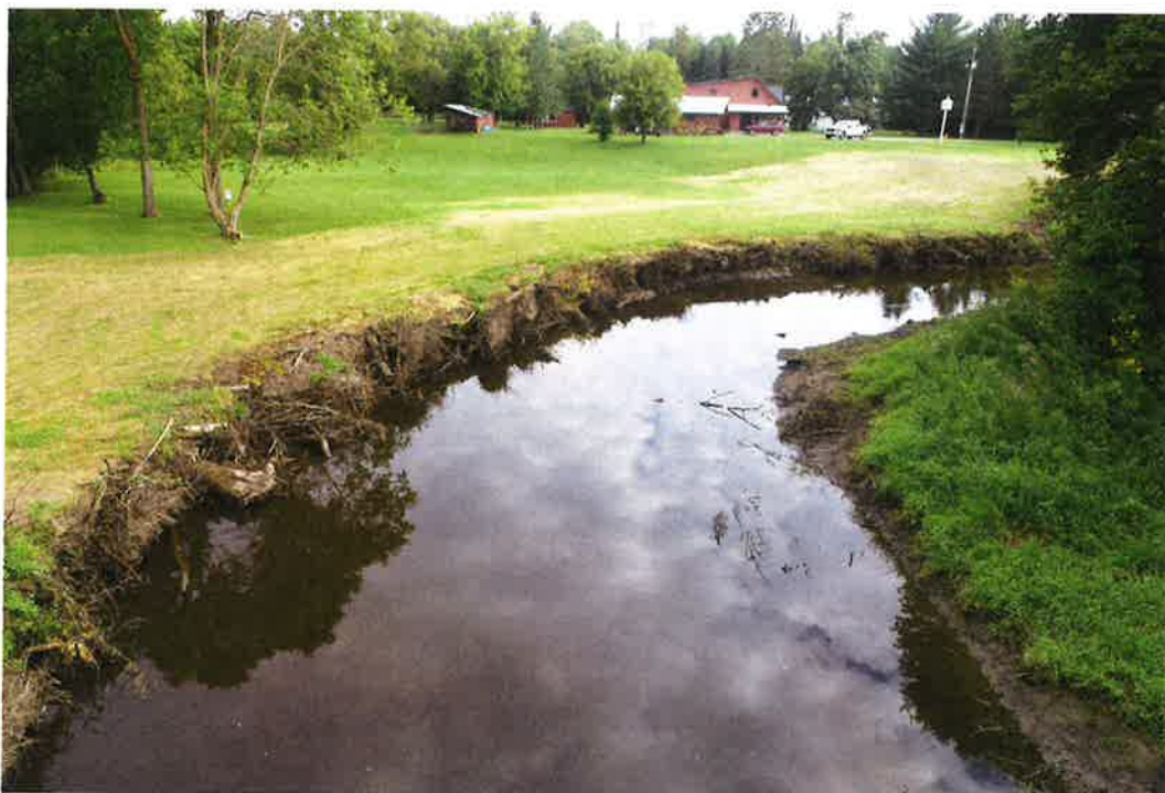
Above: Streambank stabilization project completed at the David Olson property utilizing toe wood (root ball) method of stabilization.
