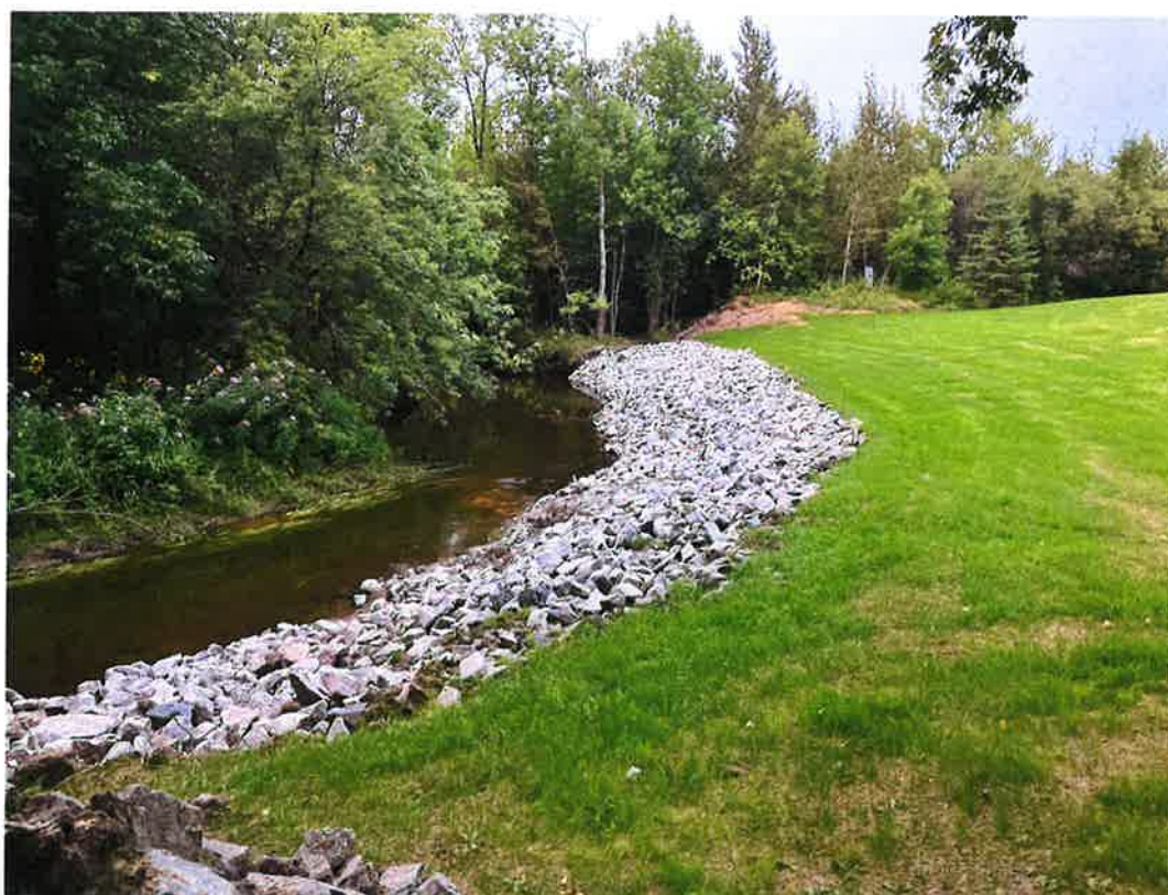
Above: Streambank stabilization project completed at the Scott Thompson property utilizing rip-rap method of stabilization.
