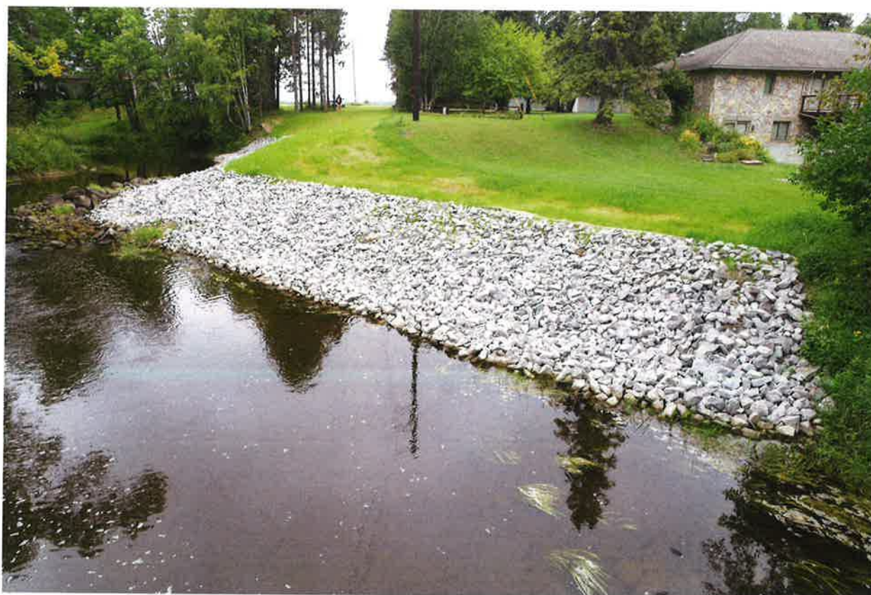
Above: Streambank stabilization project completed at the Mike and Carla Roberts property utilizing rip-rap method of stabilization.
