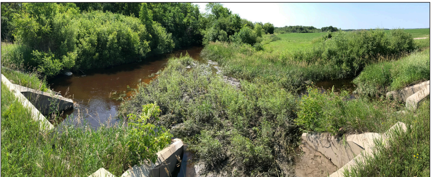
Not far from the Warroad River Watershed District project, sediment deposition was evident in culverts through which the West Branch Warroad River flowed.
