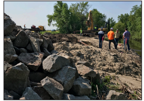
A crew from Gerit Hanson Contracting drove sheet piling into the ground in late July along the West Branch Warroad River in Roseau County. They built a 50-foot-long water control structure as part of a Warroad River Watershed District project funded by a Disaster Relief Assistance Program grant from the Minnesota Board of Water and Soil Resources. Contractors would later place rocks to help to armor the structure.
