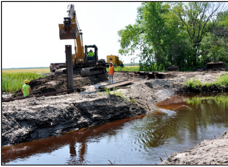
A crew from Gerit Hanson Contracting drove sheet piling into the ground in late July along the West Branch Warroad River in Roseau County. They built a 50-foot-long water control structure as part of a Warroad River Watershed District project funded by a Disaster Relief Assistance Program grant from the Minnesota Board of Water and Soil Resources. Contractors would later place rocks to help to armor the structure.
